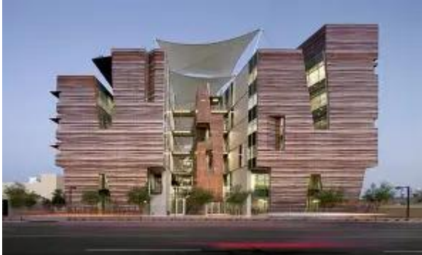
Arizona Biomedical Campus – Phoenix, USA
